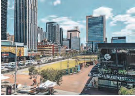
View from Yagan Square, on the outskirts of the Perth CBD © Photo by Joshua Leong on Unsplash
