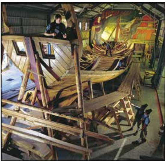
Building the Duyfken Replica Photo: Robert Garvey
